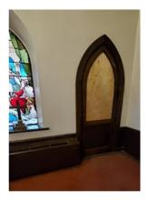
Meanwhile, inside the church, work has started on the side door located in the memorial chapel, in the area next to the organ. Lamb Studios, which has a long history with Bethesda, removed the glass from the door and transported it back to their facilities for restoration. A temporary plywood insert was installed, and the beautiful wooden door will be refinished.
