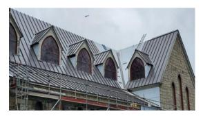
Work has progressed nicely with the addition of metal roofing on the western side of the church.
